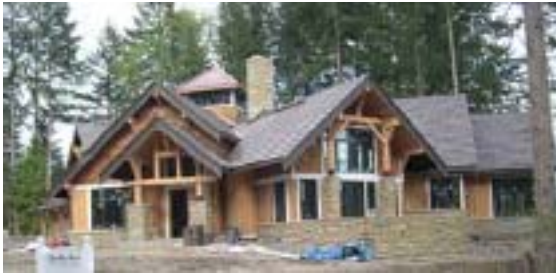
Tamarack Lodge under construction
